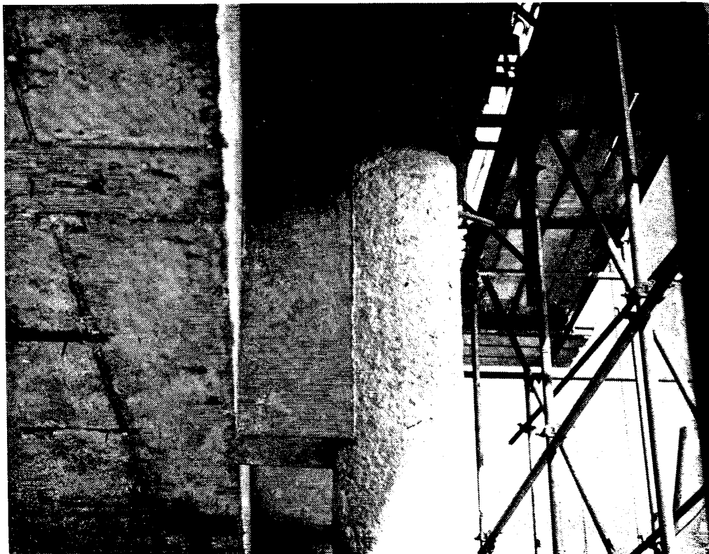
49 Supporting Precast Column Underside of typical ward floor parapet and cill showing supporting precast concrete column.
