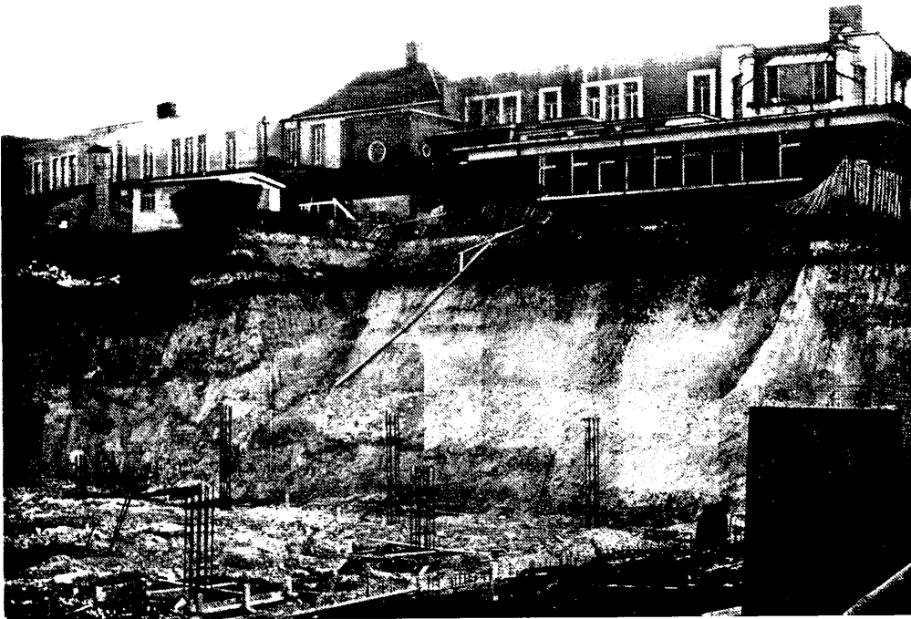
47 Excavations for Phase 1B No shoring was used for the deep excavations in chalk for Phase 1B. The old hospital building is seen above the excavations.
