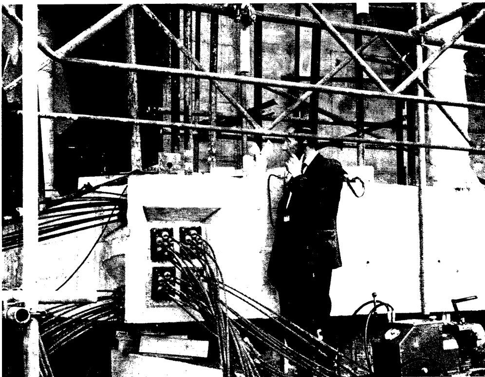
48 Corner of Prestressed Concrete Ring Beam Corner of the prestressed ring beam at 1st floor level during stressing.
