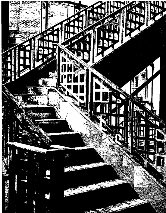
A lattice work staircase with numerous surfaces to be cleaned
