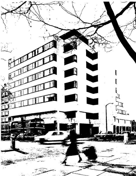
Wellington Hospital (North) – Front elevation
