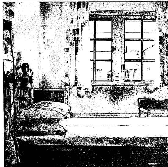
Attractive cottage style windows – but much too high if you are stuck in bed
