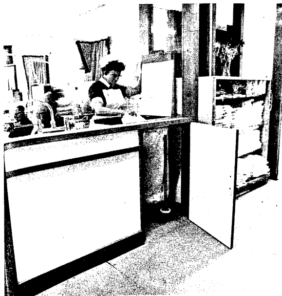
64 Greenwich—the dirty linen hatch with rounder in position.
